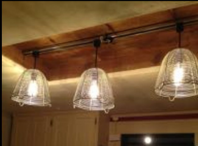
Now pendant lighting replacing recessed florescent panel now lined with reclaimed plank flooring
